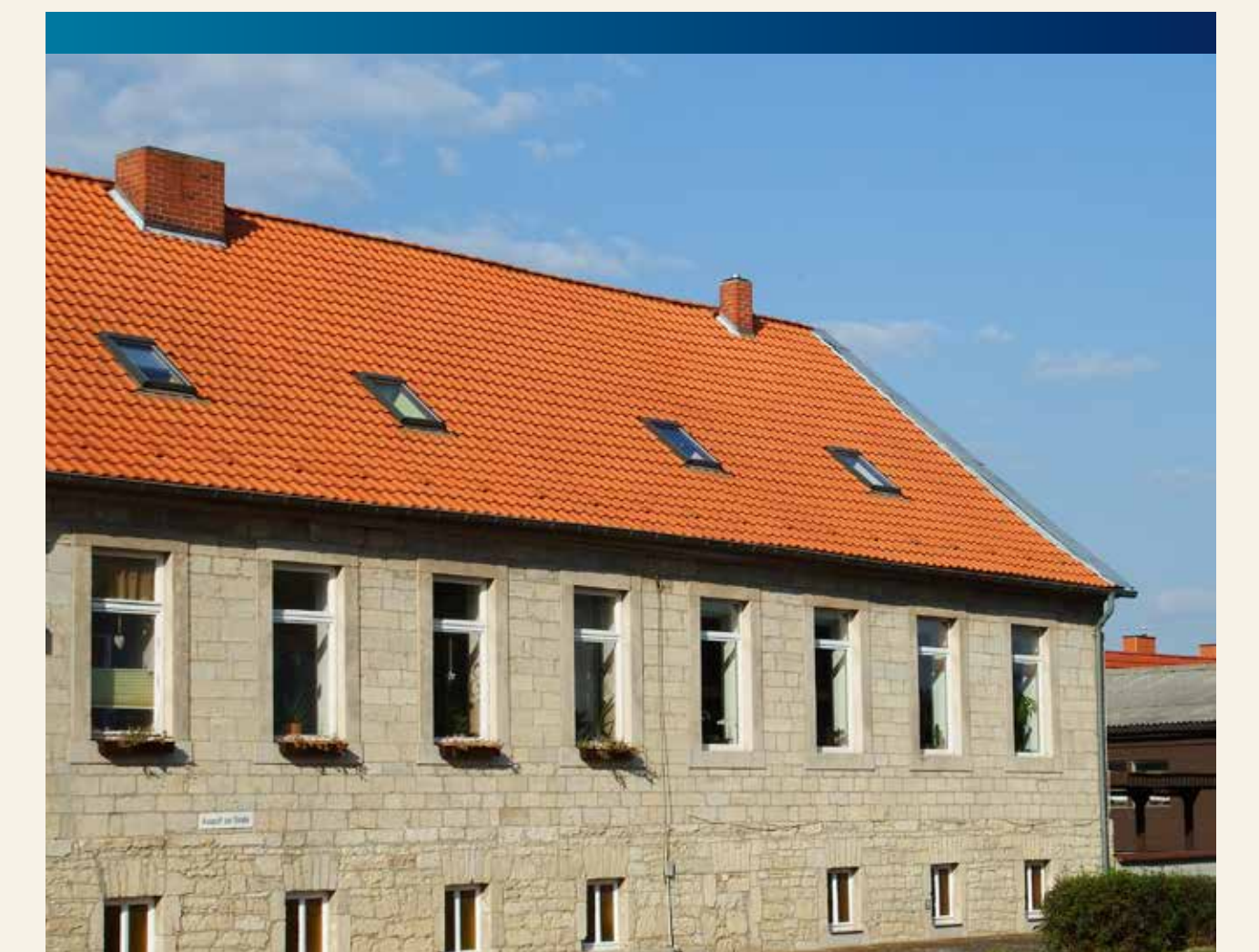
... and a secular building constructed of Muschelkalk limestone.
